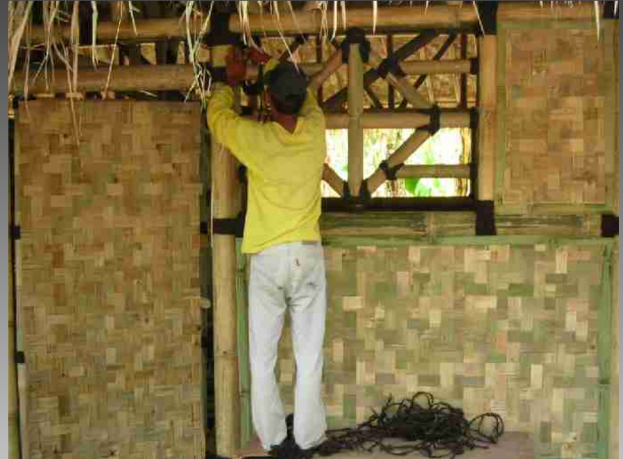
Constructing temporary schools using Bamboo, Indonesia
